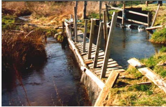
Figure 3a: Old screening arrangement at Rothiemurcus fish farm, River Spey (C1Spey12).
