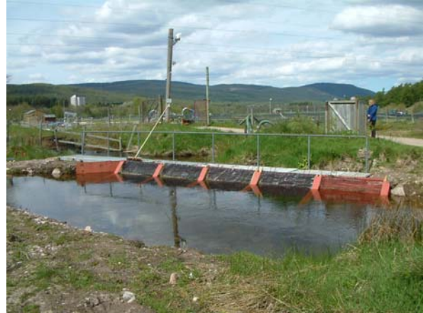
Figure 3b: New smolt screens at Rothiemurcus fish farm, River Spey (C1Spey12).
