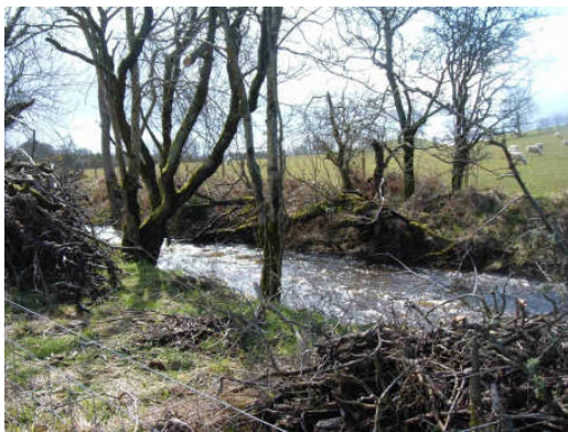
Large debris blockages on the Clugston burn have been removed to allow fish access
