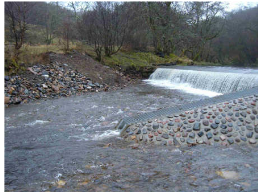
Entrance to the new fish pass fitted at Dufftown weir
