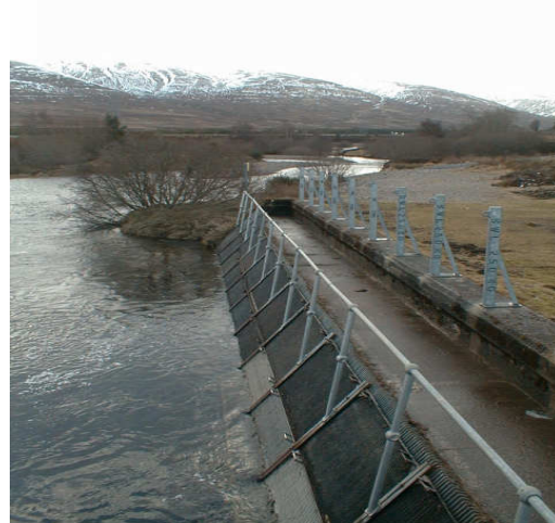
Upgrading of passage facilities and screening for salmon at man-made barriers are planned (example of screens prior to refurbishment – image courtesy of SSE)
